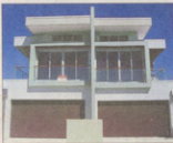
Steel frames have been used in the building of townhouses at Biggera Waters
